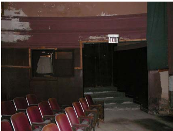
Exit alcove at west side of auditorium adjacent to stage
