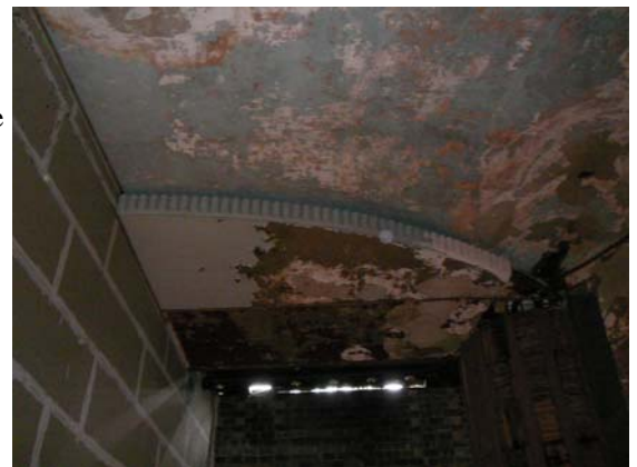
Arched soffit with sound blocks at edge of proscenium
