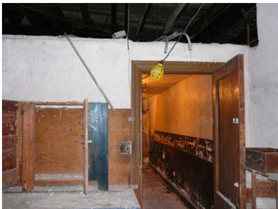
4. Storage room at east side of mezzanine
