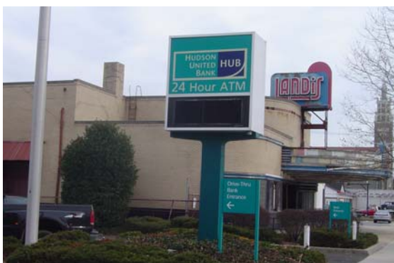
4. front portion of west façade of theatre
