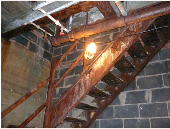
1. Metal stair from basement
