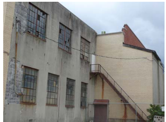
5. North façade of Mori building with exterior stairs
