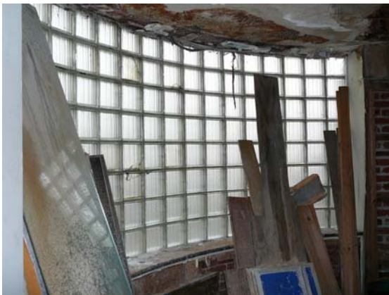
Curved glass block wall at lounge
