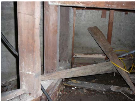
Exposed wood framing at vertical assemblies flanking stage
