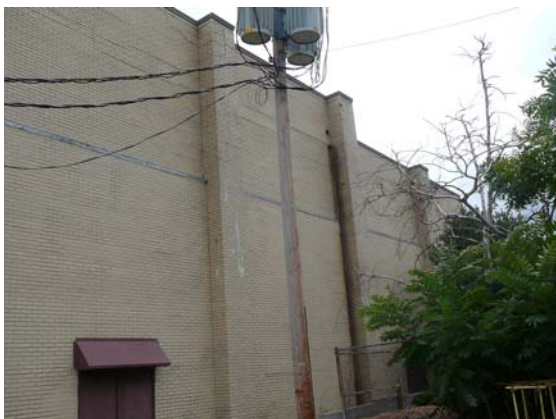
2. Rear of west façade of theatre
