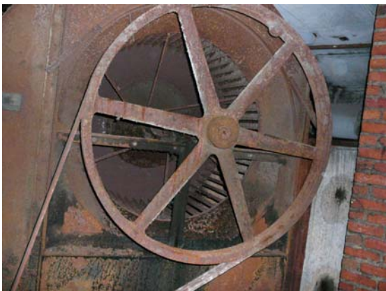
4. Portion of original mechanical system
