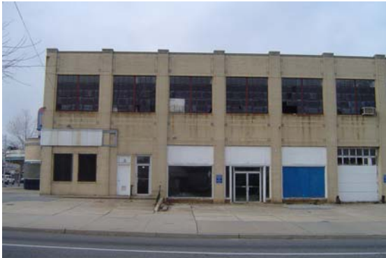
2. Southern portion of east facade
