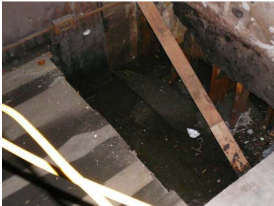
View of steps and exposed brick at vertical assembly
