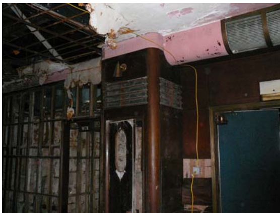
Original telephone booth at east side, note exposed framing
