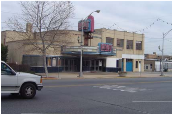
1. Southwest view of building
