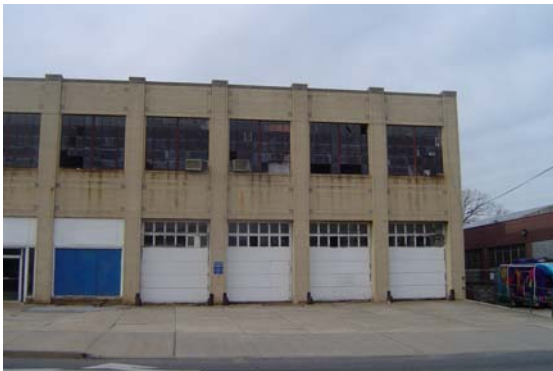
3. Northern portion of east facade
