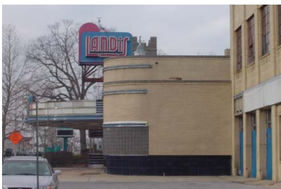
4. Side view of theatre showing curved walls and glass block
