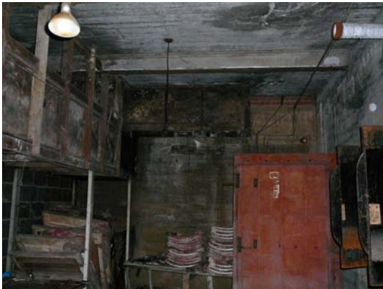
2. Upholstery area adjacent to electrical room, door to right
