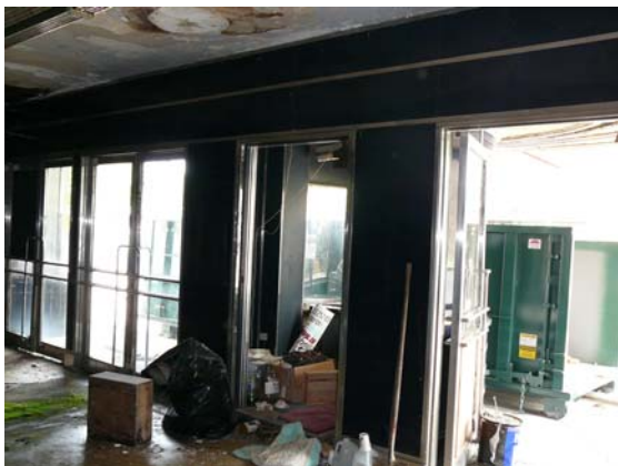
Exterior metal and glass doors and door to ticket booth
