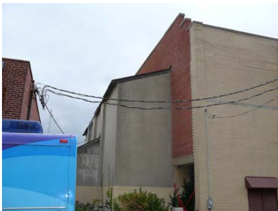
1. North façade of theatre showing stage with shed roof
