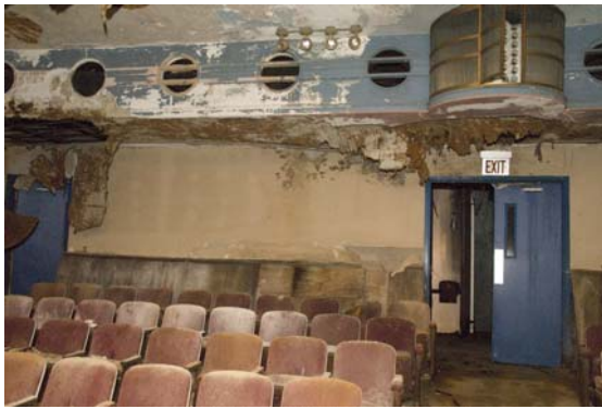
One of four glass bar light fixtures at rear of auditorium
