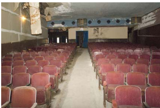
West auditorium with fifth build demising wall at left
