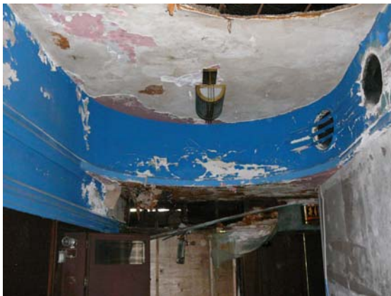
Light fixture at inner foyer, note curved plaster soffit with trim
