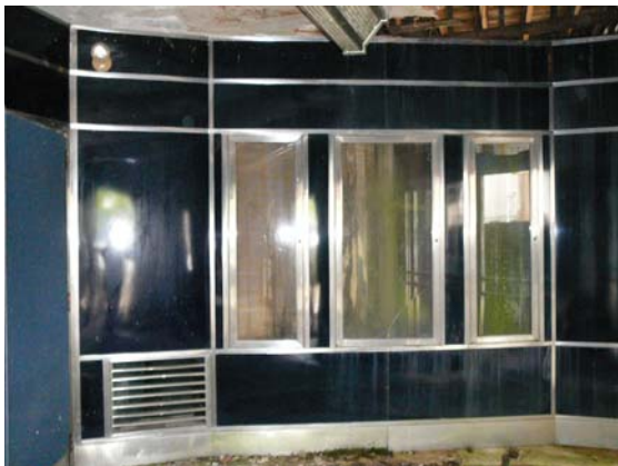
Angled side wall with display cases, note metal air register
