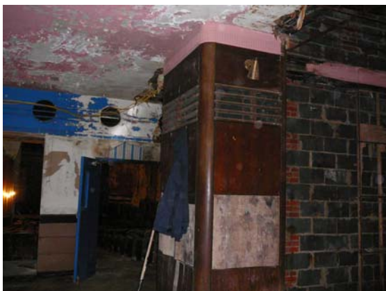
Wood veneered shaft with louver, note bare concrete walls
