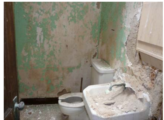
5. Employee toilet room
